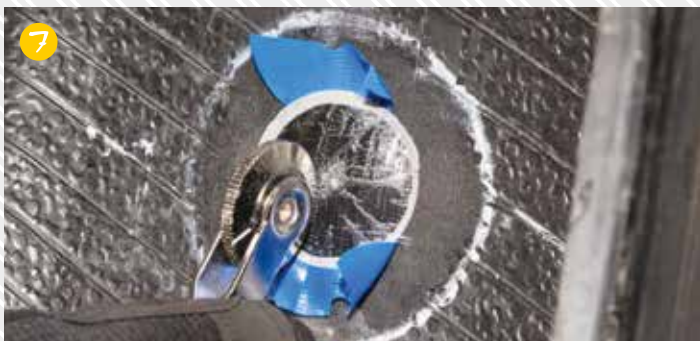
Press firmly with the roller (order no. 9245 670 029).
